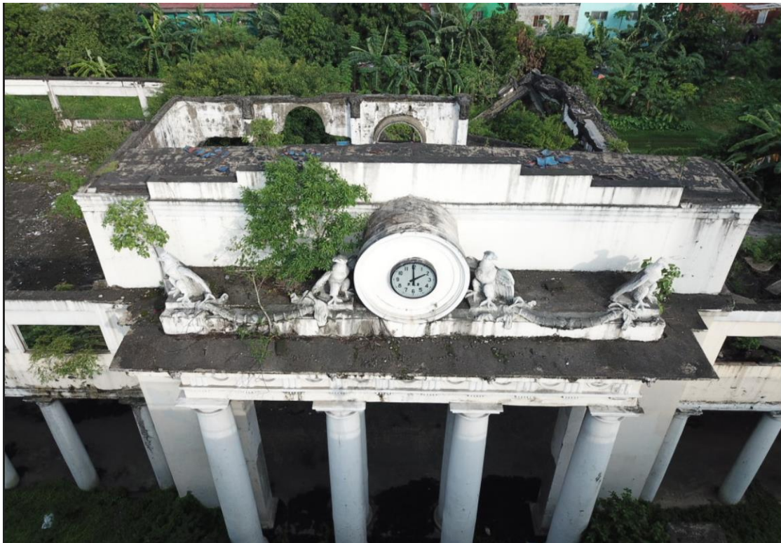
Bird's Eye View of the Facade
